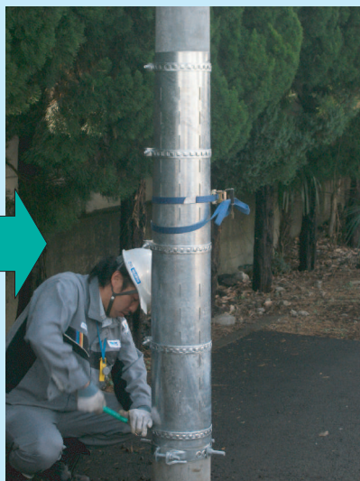
②補強板を電柱に取付け
