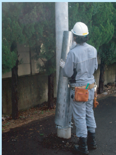
②補強板を電柱に取付け
